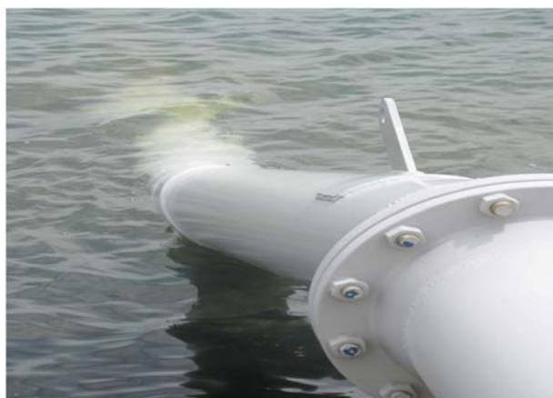
Image 1, 2, & 3: 12" pipe and drums (located adjacent to four brine pits) were treated with CleanWirx, and coated with standard epoxy coating. Equipstar storage facility maintenance project conducted in October 1995 has enjoyed over ten years of maintenance-free durability. This photograph was taken in October 2005. Project demonstrated no corrosion and no coating deterioration. Source: CleanWirx (2006).
