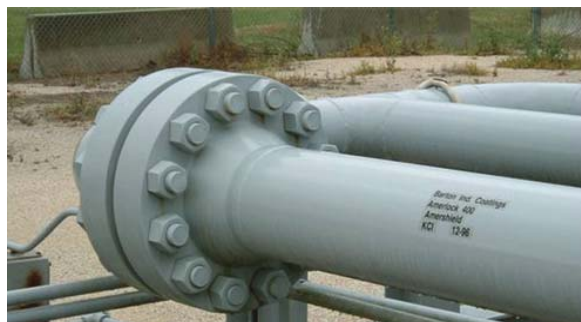
Image 1, 2, & 3: 12" pipe and drums (located adjacent to four brine pits) were treated with CleanWirx, and coated with standard epoxy coating. Equipstar storage facility maintenance project conducted in October 1995 has enjoyed over ten years of maintenance-free durability. This photograph was taken in October 2005. Project demonstrated no corrosion and no coating deterioration. Source: CleanWirx (2006).
